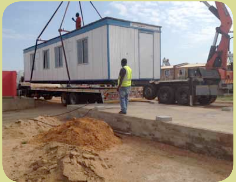
The massive structure is placed in situ
